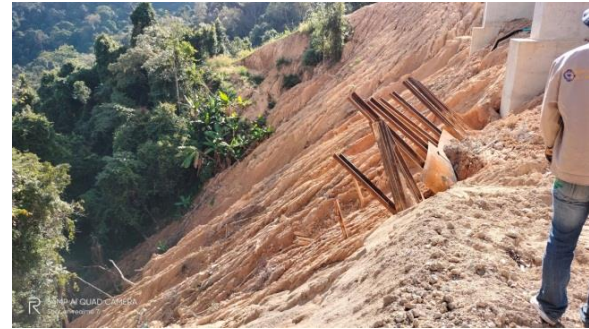
Figure 7. Show the area and nature of the failure of a slopes in Highway No.1263, section Khun Yuam - Pang Ung, at about 18+580 km LT.
