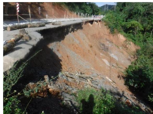
Figure 8. Show the area and nature of the failure of a slopes in Highway no. 108, section Mae Rid Bridge-Huai Ngu at km. 158+865 - km.158+923 RT.
