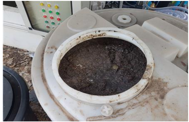
Figure 2. Polluted canal water and septic tank sludge (cont.)
