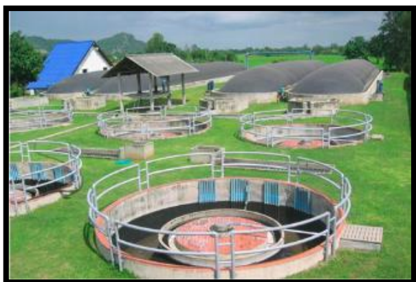
(a) Biogas system enables biogas recovery and organic fertilizer to treatment organic solid waste from biogas process.
